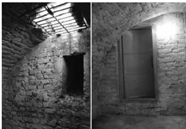
Fig. 5. The basement of Michalewski's pharmacy
